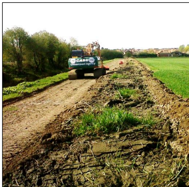
Winterton Beck: Left photo shows trench dug ready for the silt/right photo shows the trench full with silt
