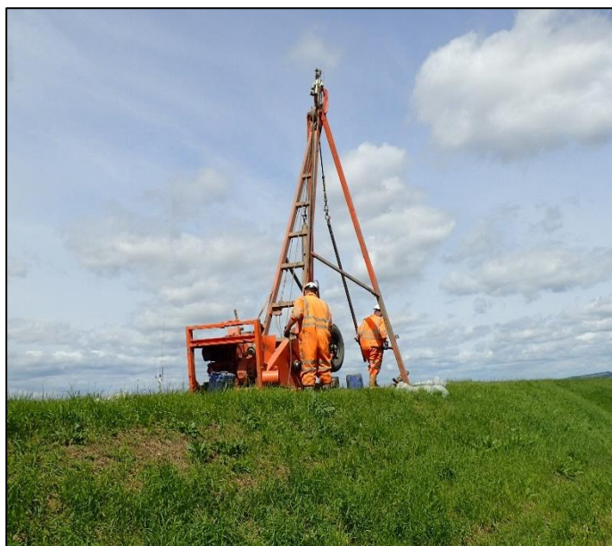
Borehole drilling on South Ferriby's flood embankments
