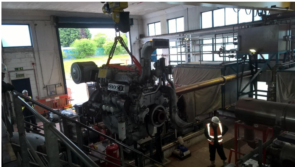
Keadby pumping station: pump engine being removed prior to its replacement
