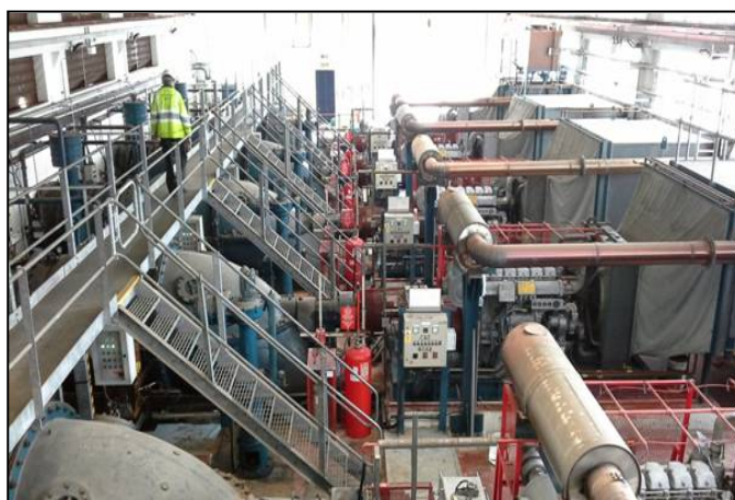
Pumps inside Keadby pumping station
