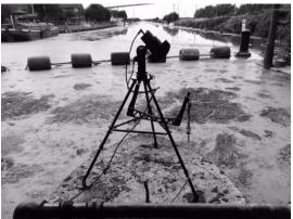
Our Operations teams have successfully de-silted 3 km of the West Drain, removing as much as 2 metres depth of silt in places. De-silting began at Ferriby Sluice and continued inland to Scabcroft Weir. De-silting the channel will increase channel capacity along the river.
