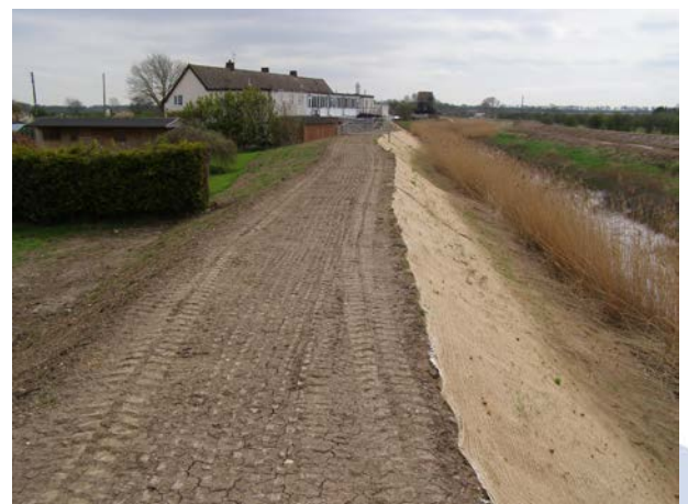
Barrow Haven: Raised low spots and widened banks.
