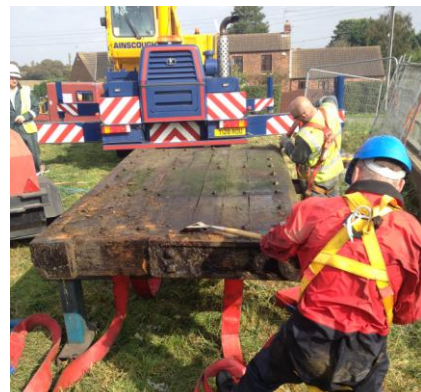
Barrow Haven: Repair works to the tidal outfall door.
