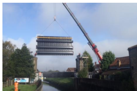
West Stockwith: Replacing the tidal gate.
