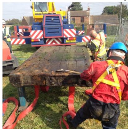
Barrow Haven: Repair works to the tidal outfall door.
